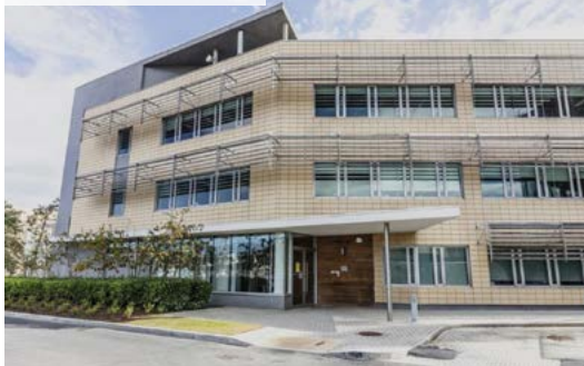
Building 8 – Dublin – Irlande
